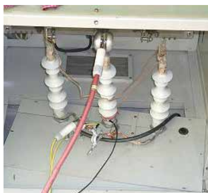
➤ Full cable not accessible, application of Expert mode enables the safe cable identification.
