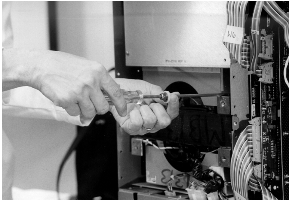
Figure 4.49 Guiding the Transformer Mounting Nuts into Position
