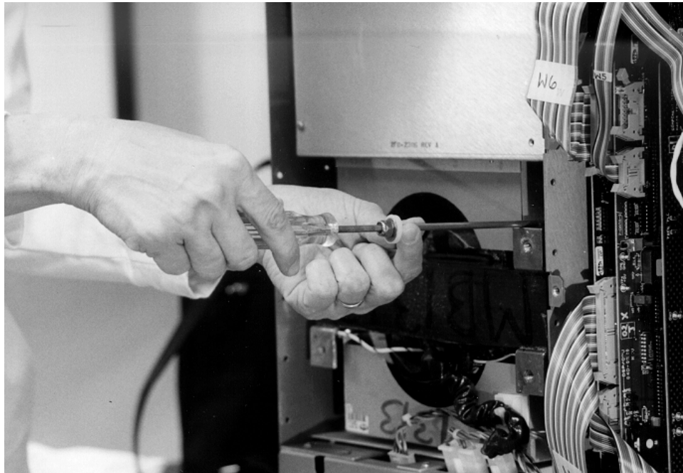
Figure 4.49 Guiding the Transformer Mounting Nuts into Position
